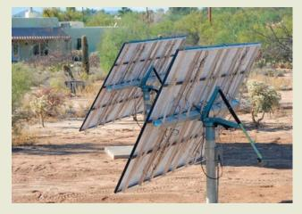
A pair of 2,720 W pole-mounted, tracked arrays at the Tucson site have generated even more energy than originally predicted.
