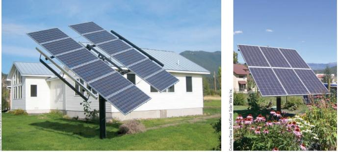
Left: A Zomeworks single-axis tracker with its outboard Freon vessels. Right: A Wattsun tracker (note the optimal sensor in the upper left corner of the array).
